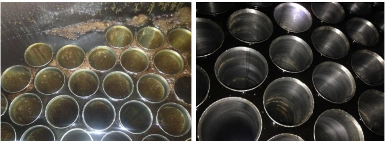
**Heating tubes showing before & after treatment using SSS international<sup>SM</sup> Treatment systems**
